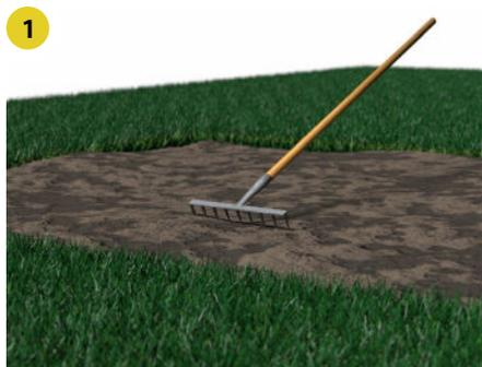
**1** **Level the garden site. This step is VERY IMPORTANT. If the site is level, installation will be MUCH FASTER.** Remove rocks, roots and debris that may prevent the panels from sitting straight and level. Using a laser level to check your work can speed up this process. Compact the soil where the walls of the bed will rest.
